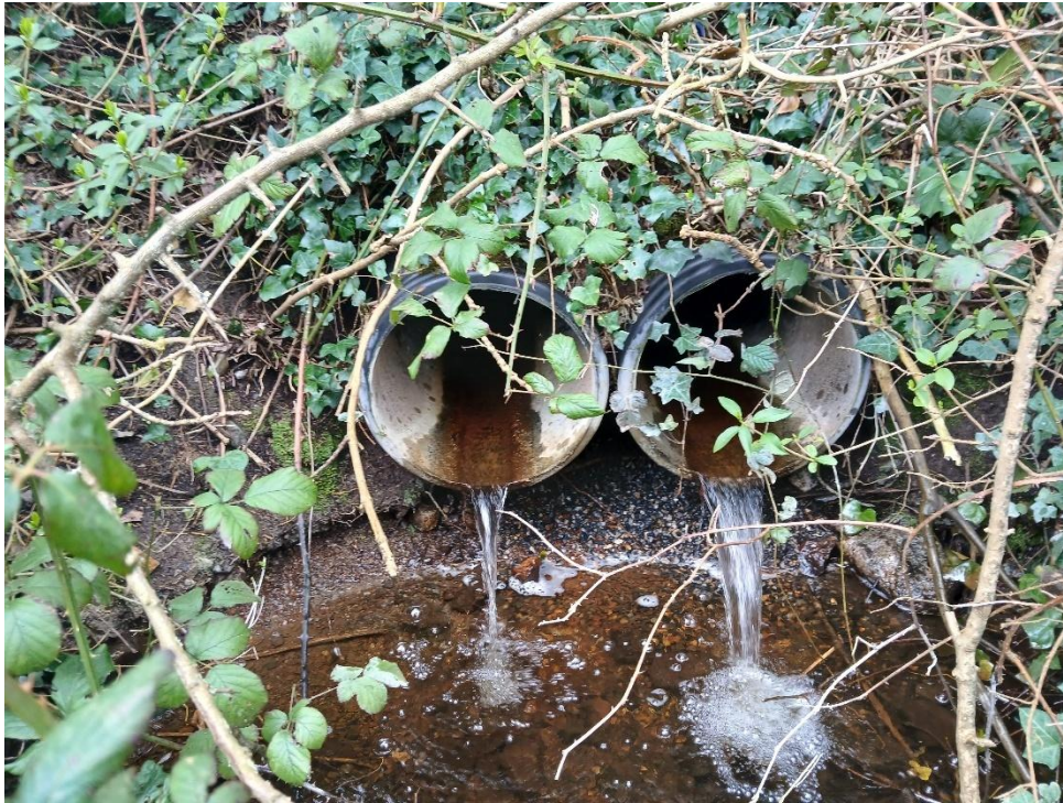
Photo 1 – Drainage pipes under local road near proposed GCR crossing location (March 2025)
